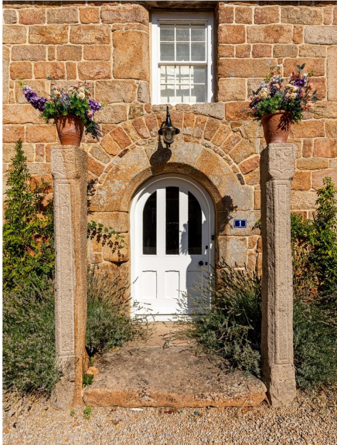
Double Voussoirs on Arched Entrance
